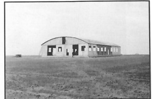
Photo taken by Gilson Wright in January 1943 of the Miami University airport's first hangar. The structure was moved from an abandoned Cincinnati airfield. Photo courtesy of the Smith Regional History Library of Oxford, Ohio.
